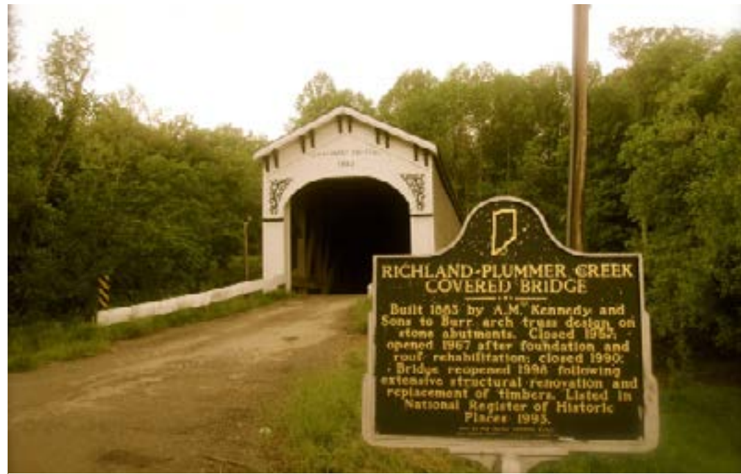
(2.) Richard-Plummer Creek Covered Bridge
